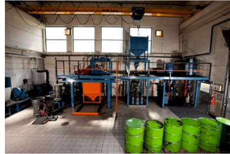
Dry aggregate preparation
