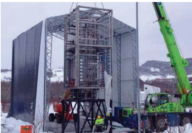
Installation of the 150 kW CLC rig. (Photo: Øyvind Langørgen)
