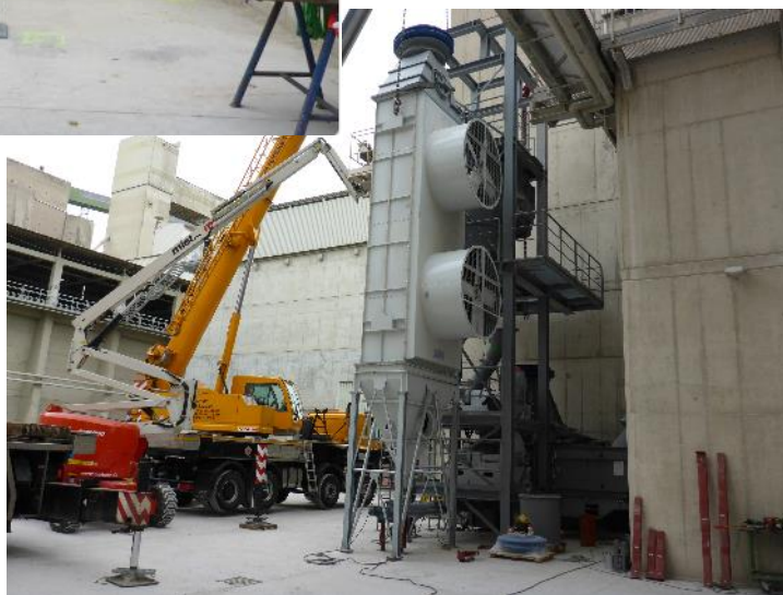
Clinker cooler prototype and recirculation system installation at HeidelbergCement in Hannover
