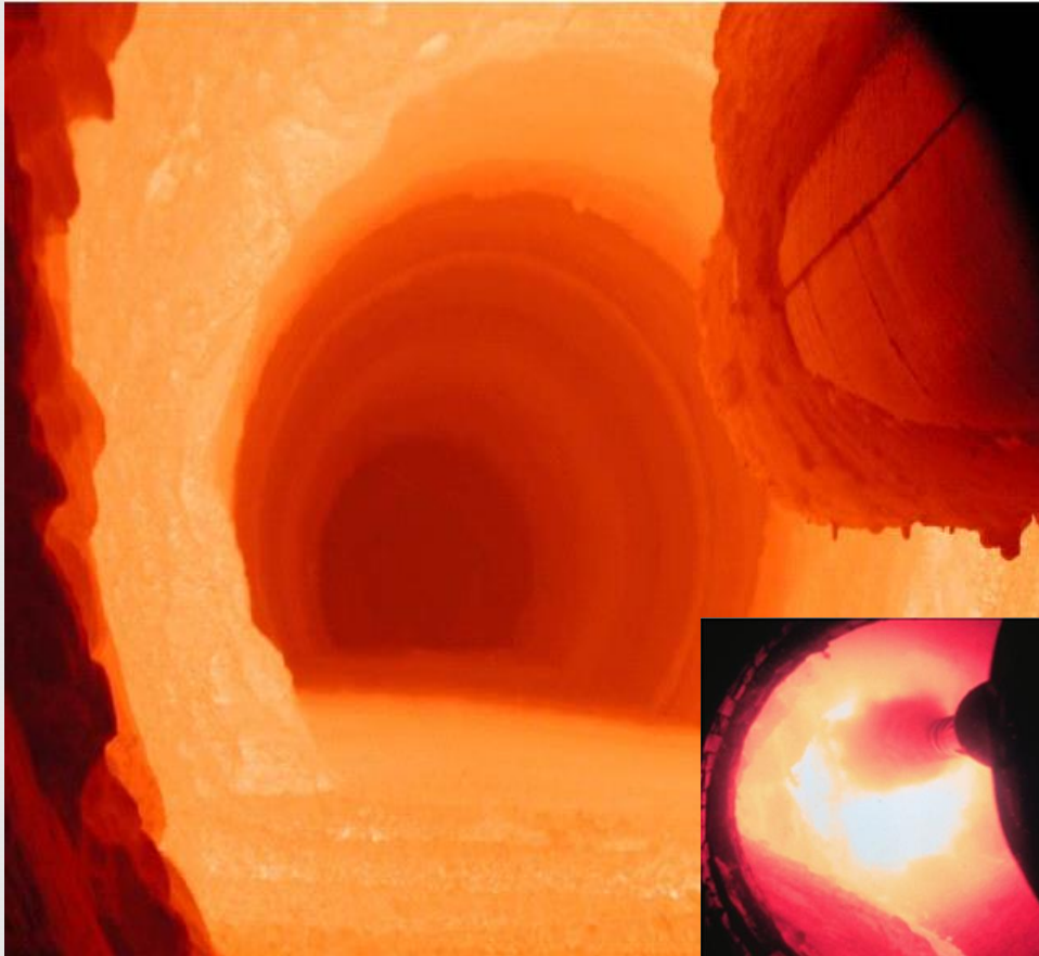
View into a rotary kiln
