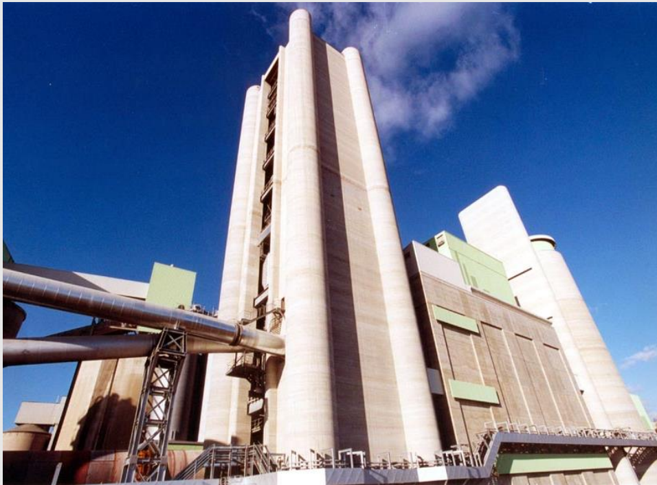
Cement plant with rotary kiln, preheater tower and raw material grinding
