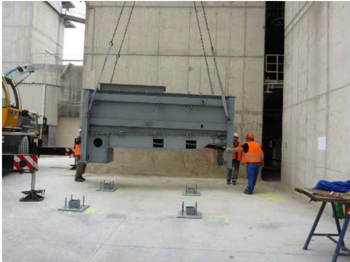
Clinker cooler prototype and recirculation system installation at HeidelbergCement in Hannover
