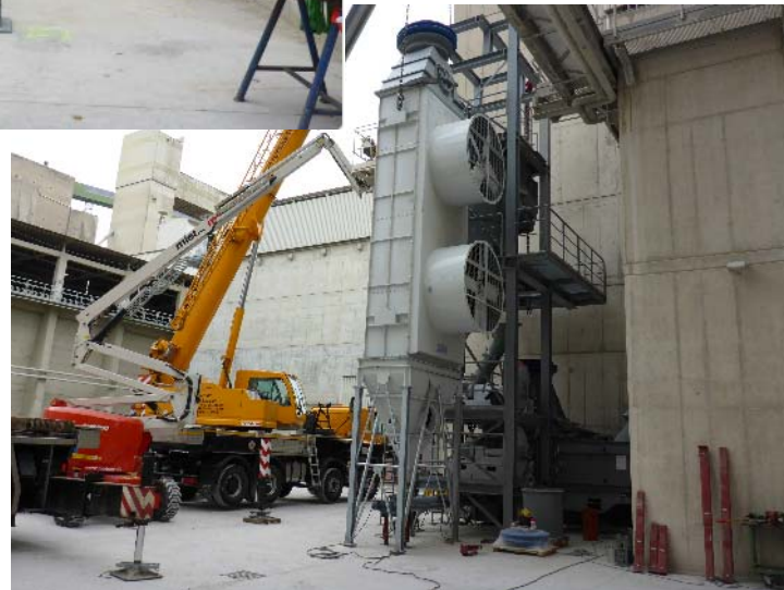
Clinker cooler prototype and recirculation system installation at HeidelbergCement in Hannover
