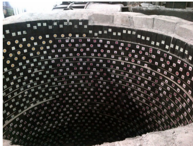
Figure 5: Ladle with freshly layed bricklining.
