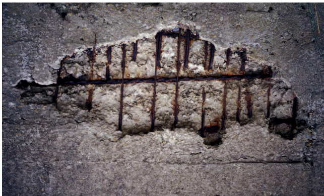
Figure 1: Corroded re-bars
