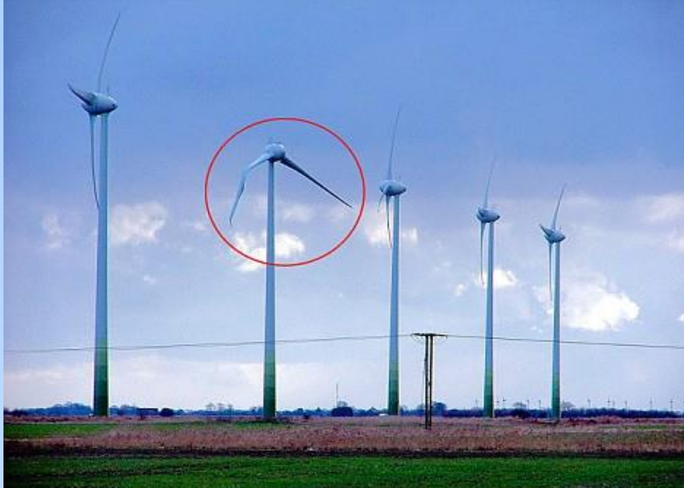
Failure of a wind turbine blade
