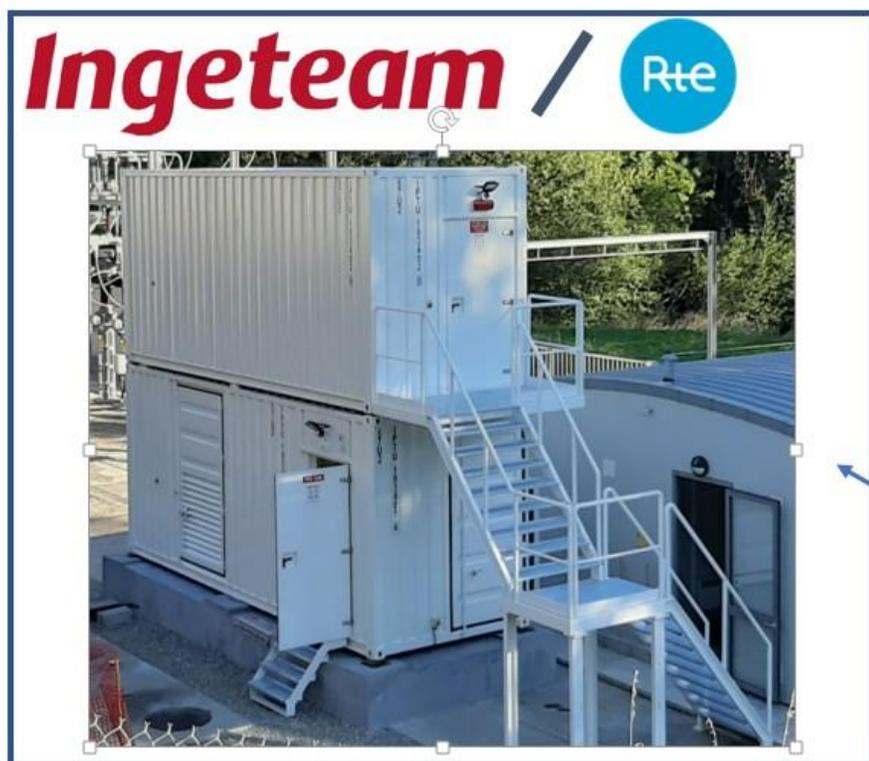
A 1 MVA solution built for the project and connected to a 20 kV feeder in a RTE substation, including
