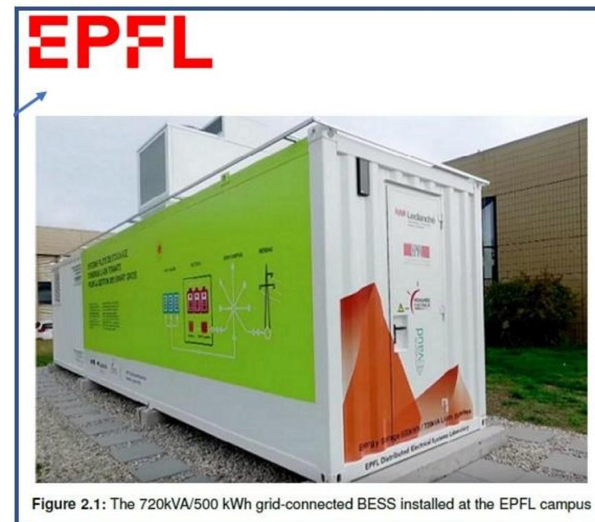
Figure 2.1: The 720kVA/500 kWh grid-connected BESS installed at the EPFL campus
