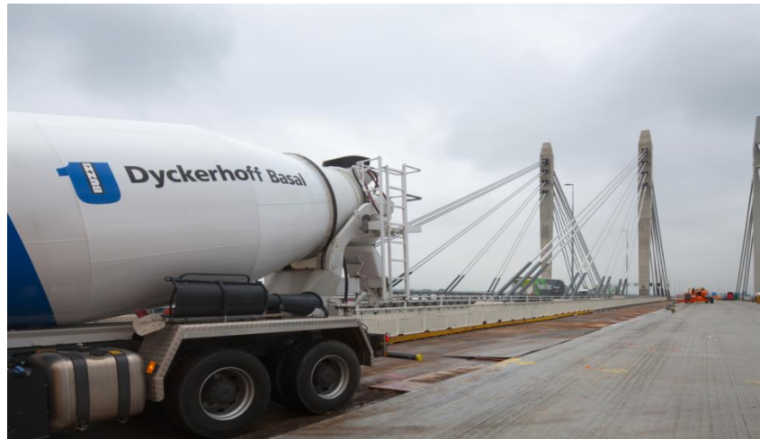
Figure 1: Dyckerhoff developed a concrete concept to meet the demanding requirements for the rehabilitation of the bridge. (Photo: Bart van Hoek)
