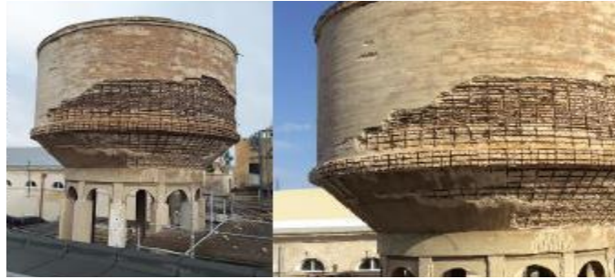
Figure 4: The steel-reinforced concrete of the water reservoir tower in the Grand Harbour region of Malta, to be retrofitted with TRC
