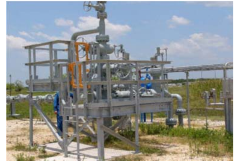
Outlet valve of a hydrogen cavern
