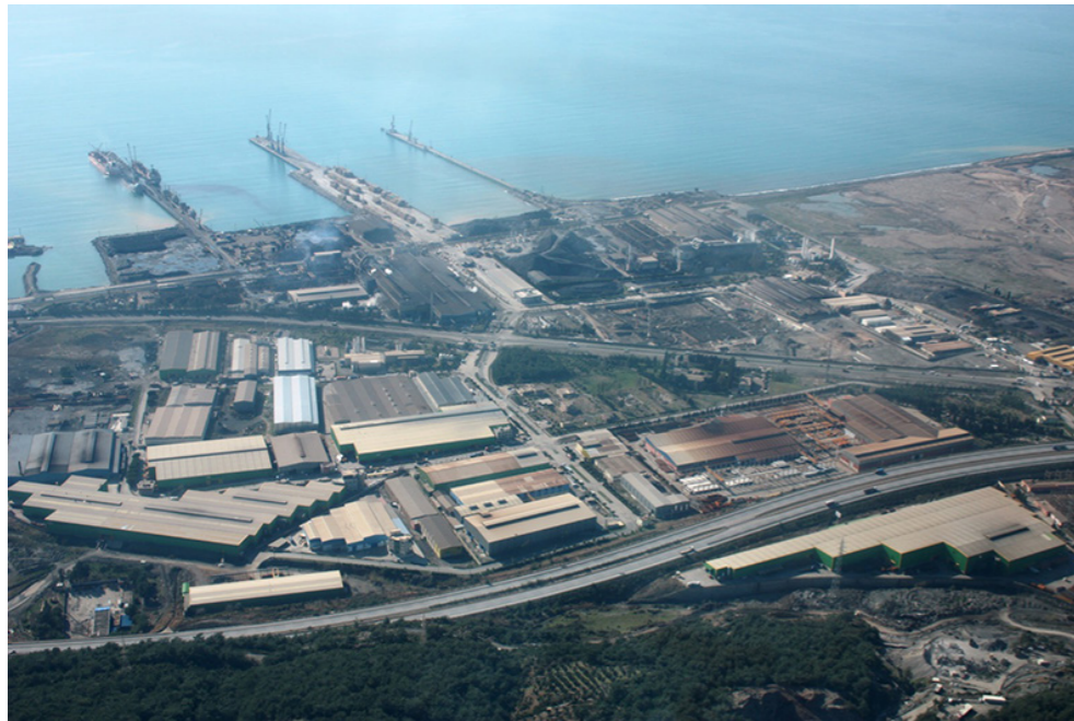
Noksel's Iskenderun Plant with annual 200.000 Tons production capacity at Hatay region in Turkey.
