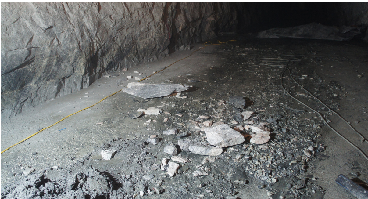
Fig. 8. Rock burst with rock fragment released.
