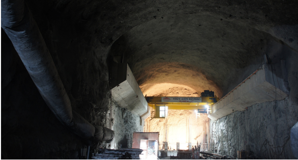
Fig. 9. Underground powerhouse cavern of the Su-Pan 1 HPP – During construction.
