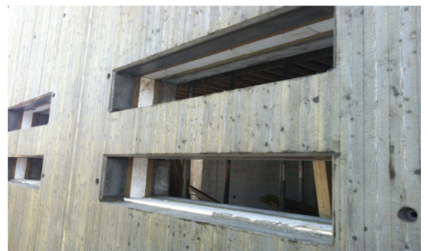
The façade walls in Veidekkes new office buildings at Rudshøgda are successfully reinforced with Basaltic fibres (Reforcetech's Minibars)
