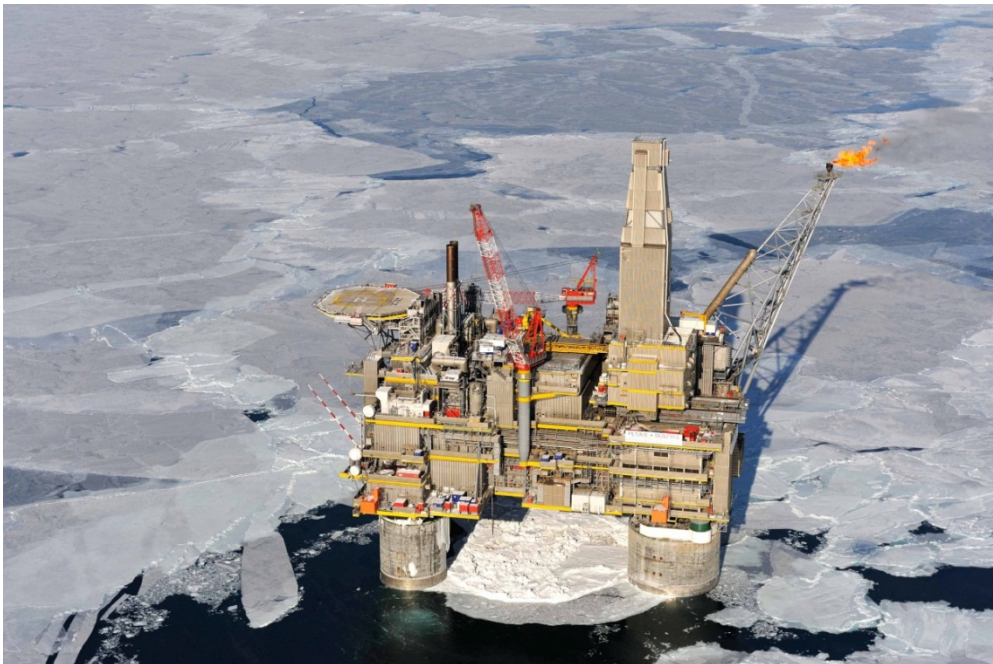
Sakhalin-2: concrete gravity base structure for the offshore platforms
