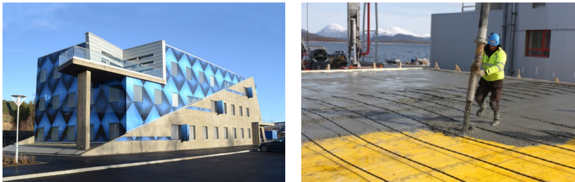
Figure 8: Reference projects (a) Veidekke's headquarter at Rudshøgda in Hedmark, and (b) Fibre reinforced post-tensioned slab in Spjelkavik.
