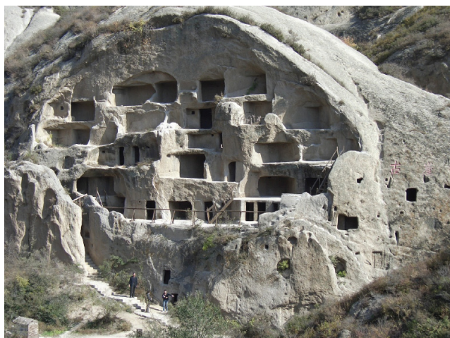
Figure 2: Utilisation of thermal mass of heavy structures, here in Guyajuruinene, China. Photo: pftcdyelise (from Wikipedia)
