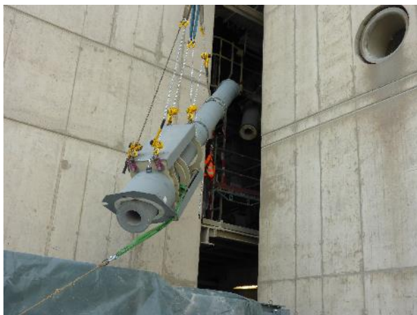
Clinker extraction device being mounted
