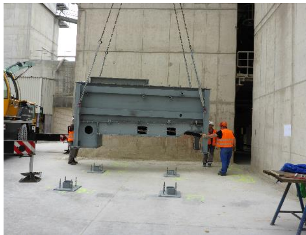
Installation of clinker cooler
