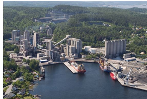
(NORCEM project in planning Photo: NORCEM)
