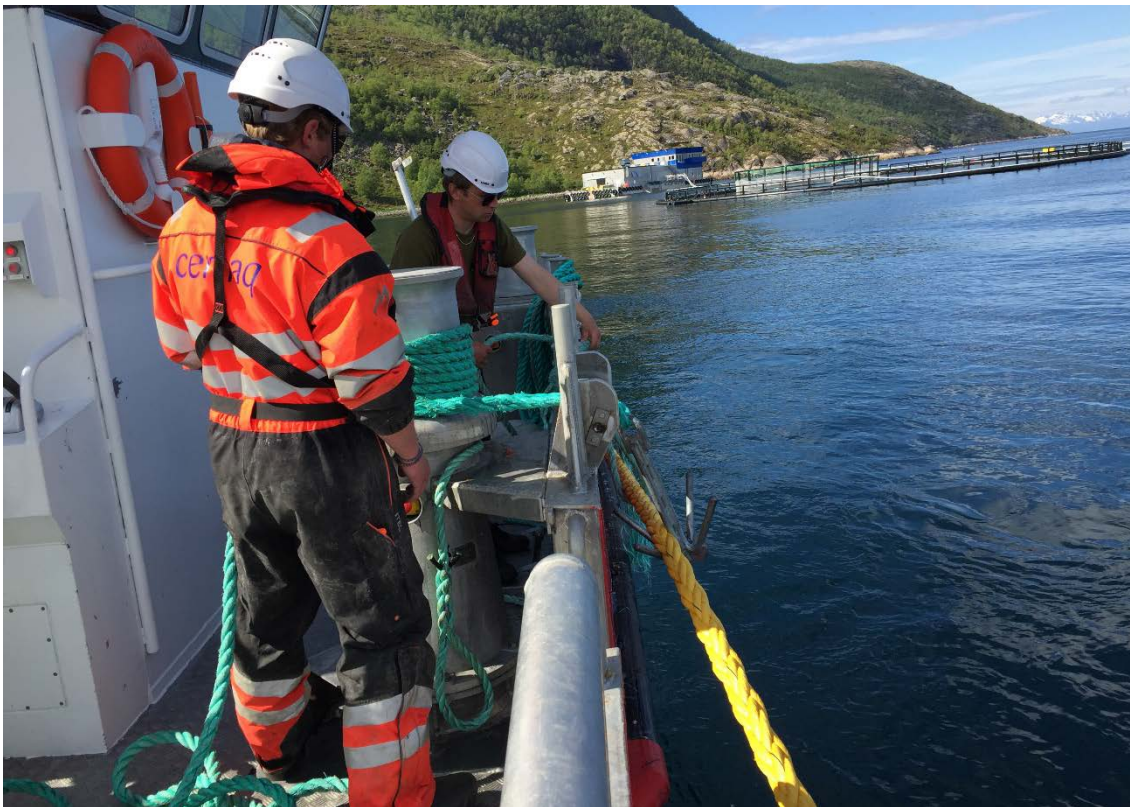
Figure 17 Maintenance work on mooring line. Photo: SINTEF Ocean (with permission from Cermaq Norway)
